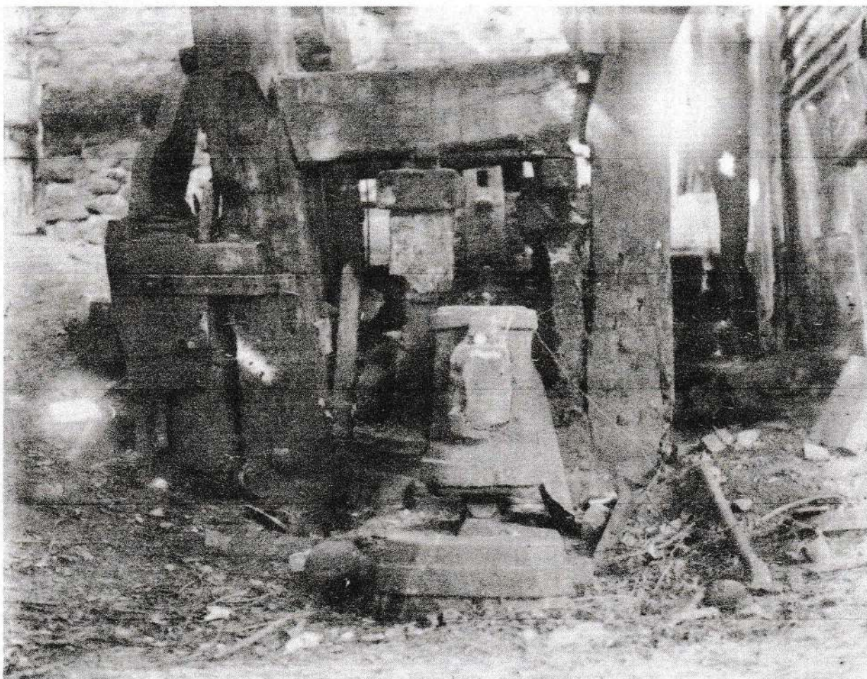
The Great Hammer at Steeds' Iron-Works
